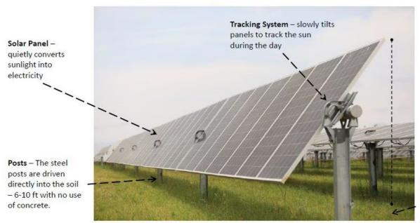
Height – Solar arrays typically stand less than 14feet high, and the site is enclosed with an 8-foot-tall safety fence
